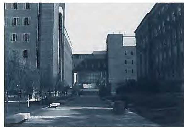
The pedestrian walk, formerly California Street. The new Chemistry Building on the right is connected via overhead walkway with the Life Science Building on the left.
